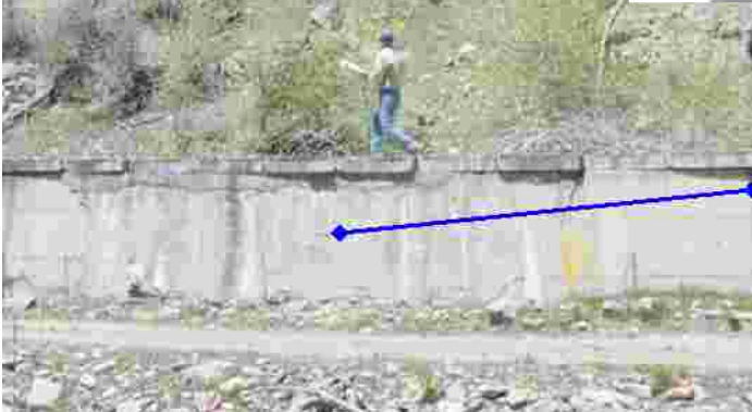
Patch in Canal Wall Due to Rock Fall
