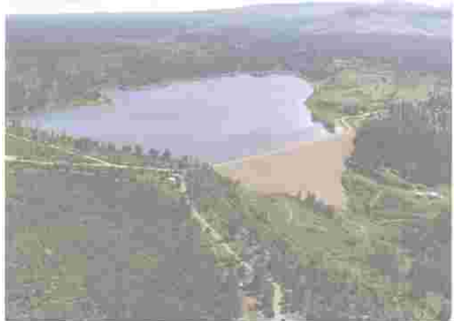
Jackson Gulch Dam and Reservoir
