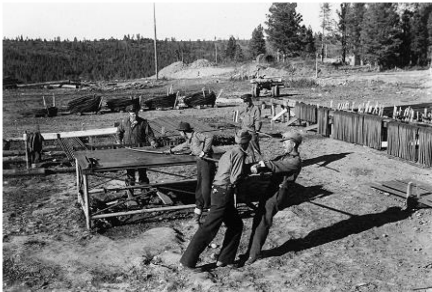
Steel re-bar bending crew. Budd Steinhilber is doing the heavy work on the bending lever (left), while the Amburgy brothers (Wayne and Claude) in the captain's hats, and others look on.
