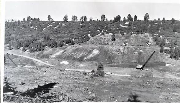
71. West abutment from photograph station 1, showing stripping work on lower toe of Jackson Gulch Dam. June 1, 1942
